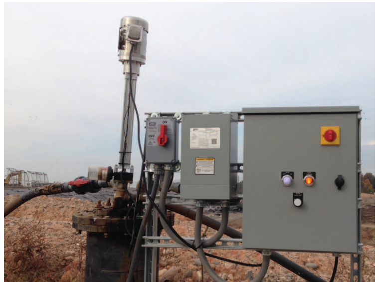
Pump controls customizable to application (Shown: Anchor Electric)
