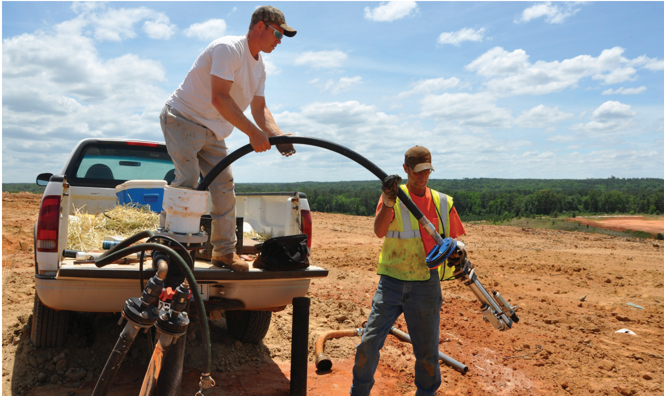
Final assembly – Slide drive rod into pump driver
