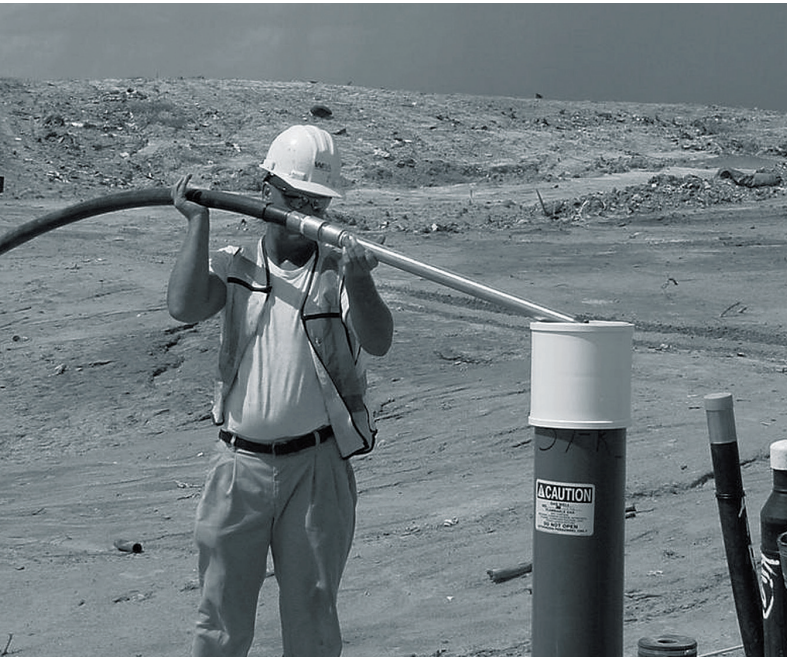
Install downhole assembly into riser pipe
